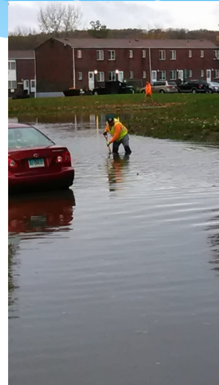
PW Utility Worker Clearing Blocked Storm Drain During Flooding
