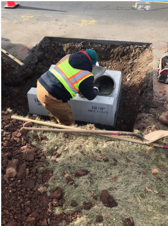
City Mason Installing New Catch Basin Top
