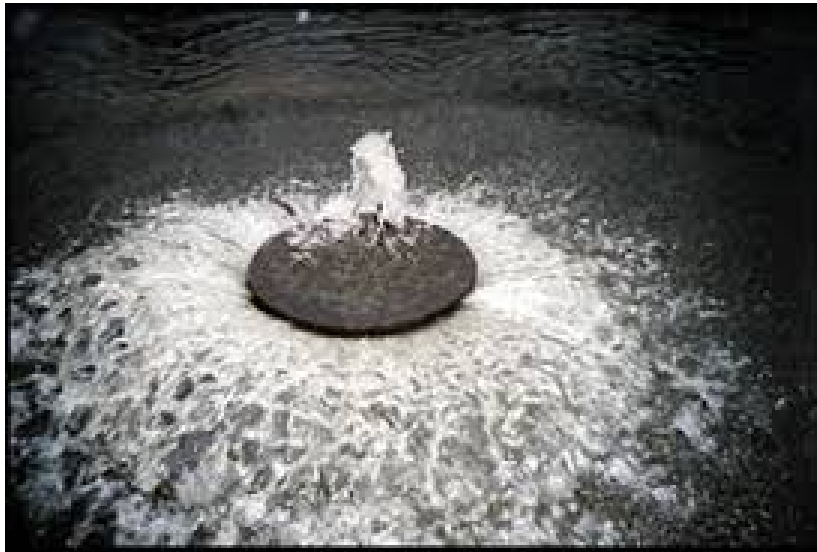
Sewer Cover Coming off due Excessive I&I
