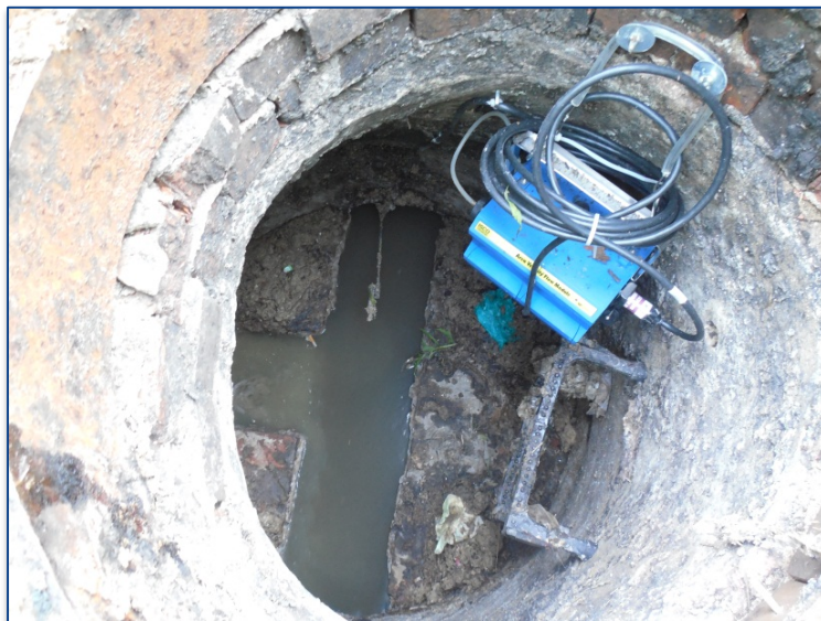
Sanitary Sewer Manhole Flow Meter
