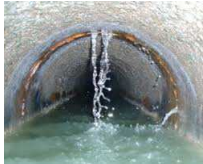
Sewer Main Infiltration
