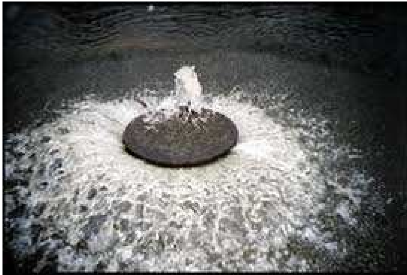
Sewer Cover Coming off due Excessive I&I
