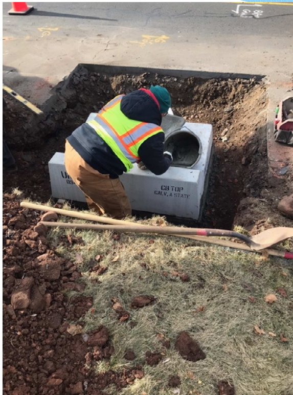
City Mason Installing New Catch Basin Top
