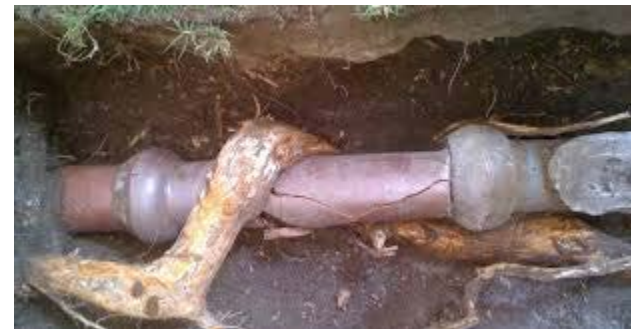
Typical Examples Sanitary Sewer System Tree Root Damage
