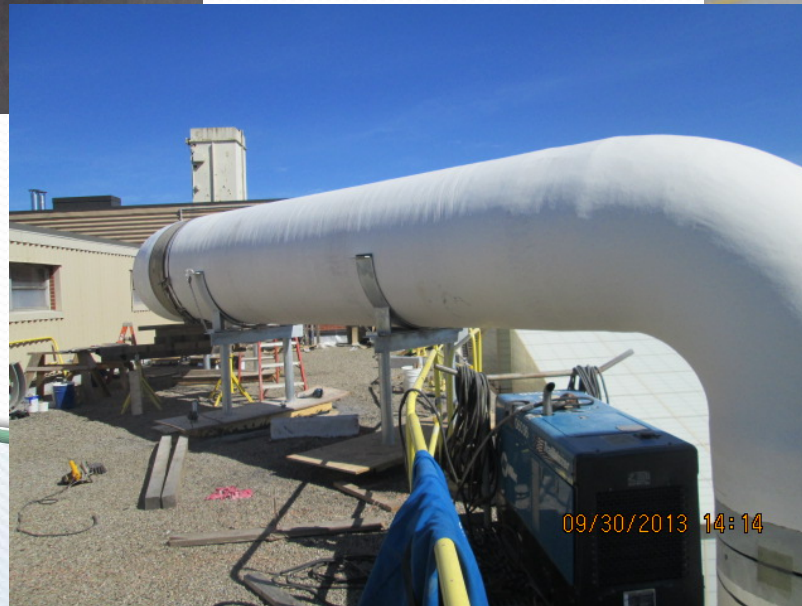
Waste Heat Recovery from Fluidized Bed Incinerator
