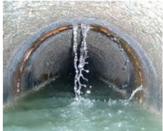
Sewer Main Infiltration
