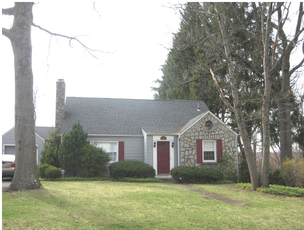
This Minimal Traditional dwelling at 100 Overhill Avenue has an exterior of both stone veneer and frame.
