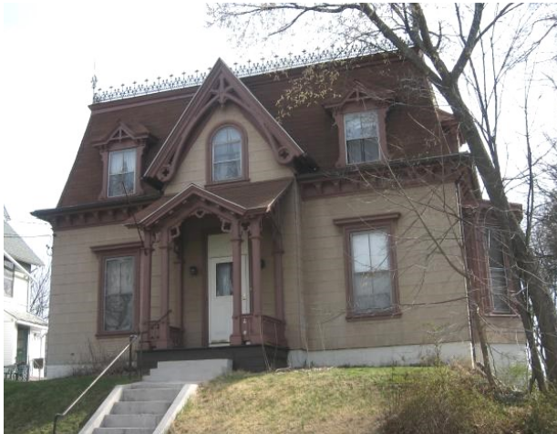
The wooden trim in the eaves, cast iron ridge cresting on the roof, additional front-facing gable, and steeply pitched roof at 101 Fairview Street all mark it as an example of the Gothic Revival style.
