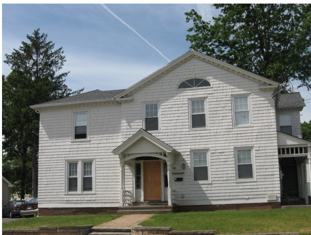
The Andrews House at 1484 Stanley Street (left) was designed in a gable front temple form and features a lunette in the gable field. Its porch and exterior shingles were added in the late 19th century.
