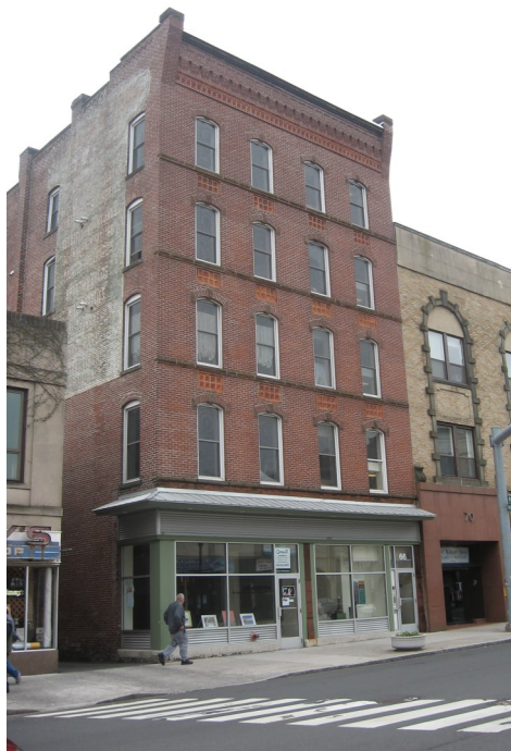
Hick's Block (Artist's Collaborative) at 66-68 W. Main Street was built in 1871 and features arched windows and a corbelled brick cornice.
