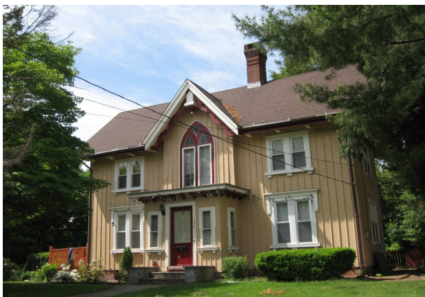
The Ethan Andrews House at 1450 Stanley Street was built with board and batten siding and a prominent central Gothic arch window.
