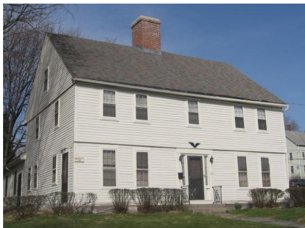
The ca. 1746 Ezra Belden House, at 639 Arch Street in the original East Street settlement cluster, demonstrates many Georgian features, including a central chimney, side-gabled roof, symmetrical five-bay façade, and central entrance.
